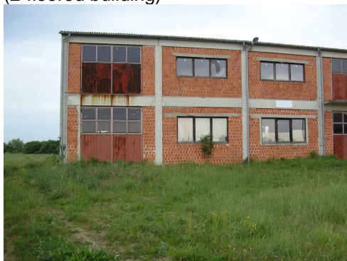
View from the access-road (2-floored building)
