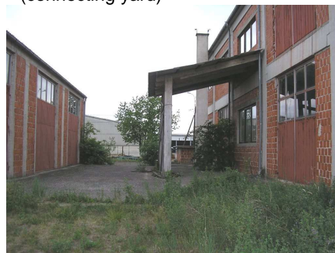
Building 1 and 2, view from the South (connecting yard)
