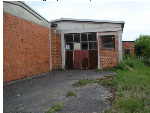
View North-West, building 2 (the wall) and building 3 (entrance)
